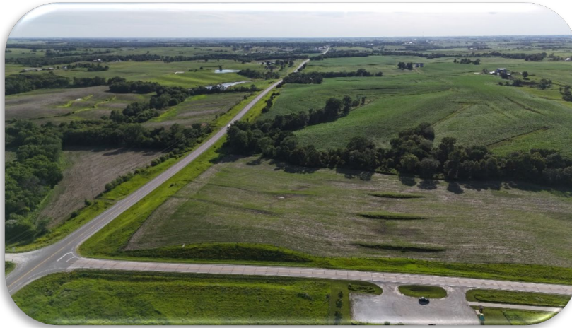
Figure 78-Aerial View of Belva Deer to Sigourney connection viewing West
