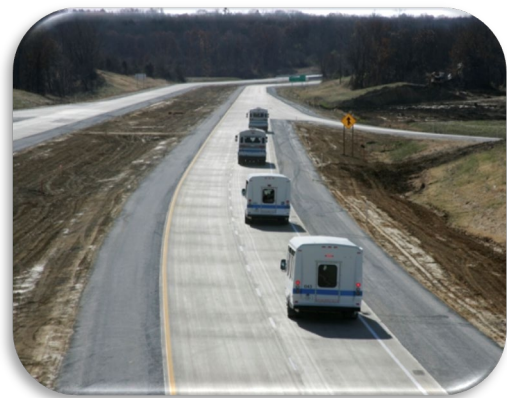
Figure 21-Transit buses along Hwy 163 near Eddyville
