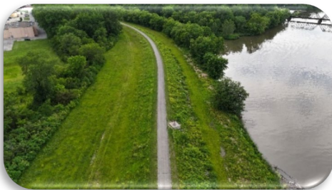
Figure 50- Aerial View of Ottumwa Trail on the levee viewing East
