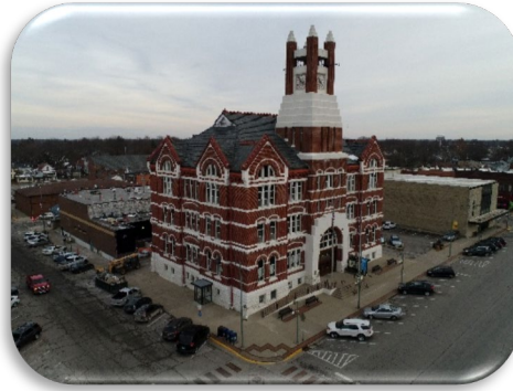
Figure 2-Picture of Mahaska County Courthouse
