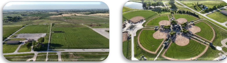
Figure 38-Figure 22- Aerial pictures Lacey Recreational complex
