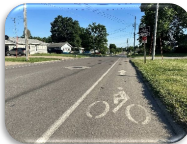
Figure 25-Bike Lane in Oskaloosa on S H St
