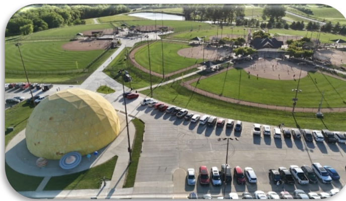
Figure 39- Aerial pictures Lacey Recreational complex
