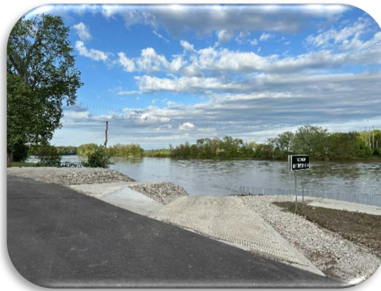
Figure 68-Lower Des Moines River Van Buren County Boat Ramp awarded by TAP funds 2026 $318,000
