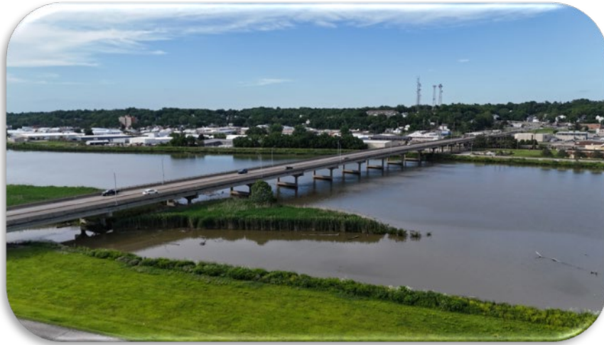
Figure 81- Hwy 149/business 63 bridge will be programed FY31 for Bridge Rehabilitation with a possible Sidepath connecting trails
