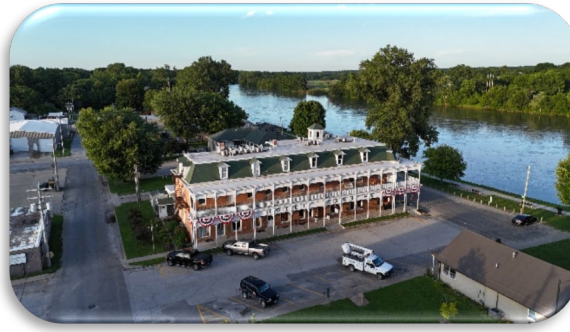
Figure 76-Aerial view of Keosauqua Manning Hotel next to the Water Trail access and Keosauqua Trail Loop
