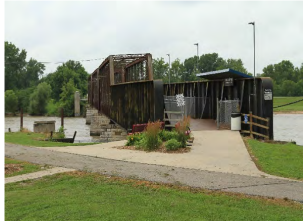
Figure 6.13: The Wabash Railroad Bridge was converted to a trail bridge and now connects the levee trails across the Des Moines River.
